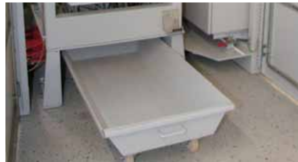
Spillage cart under the filling impeller
